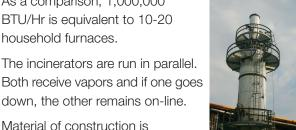
Material of construction is stainless steel to minimize corrosion.
